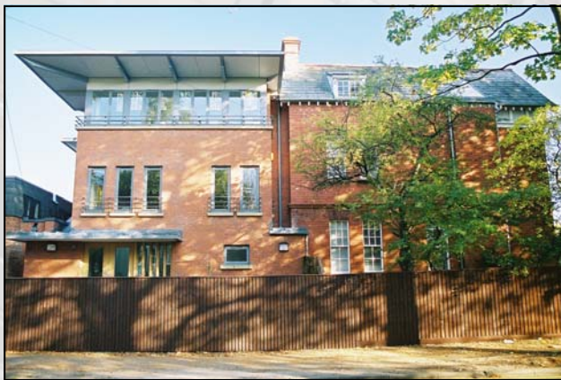
A £500k three Storey extension to Berkhamstead School, Cheltenham
